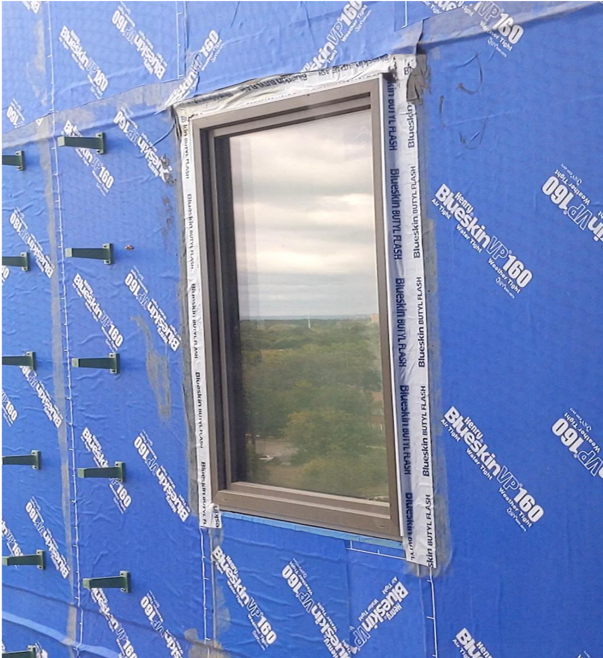
Leak detection with smoke testing
