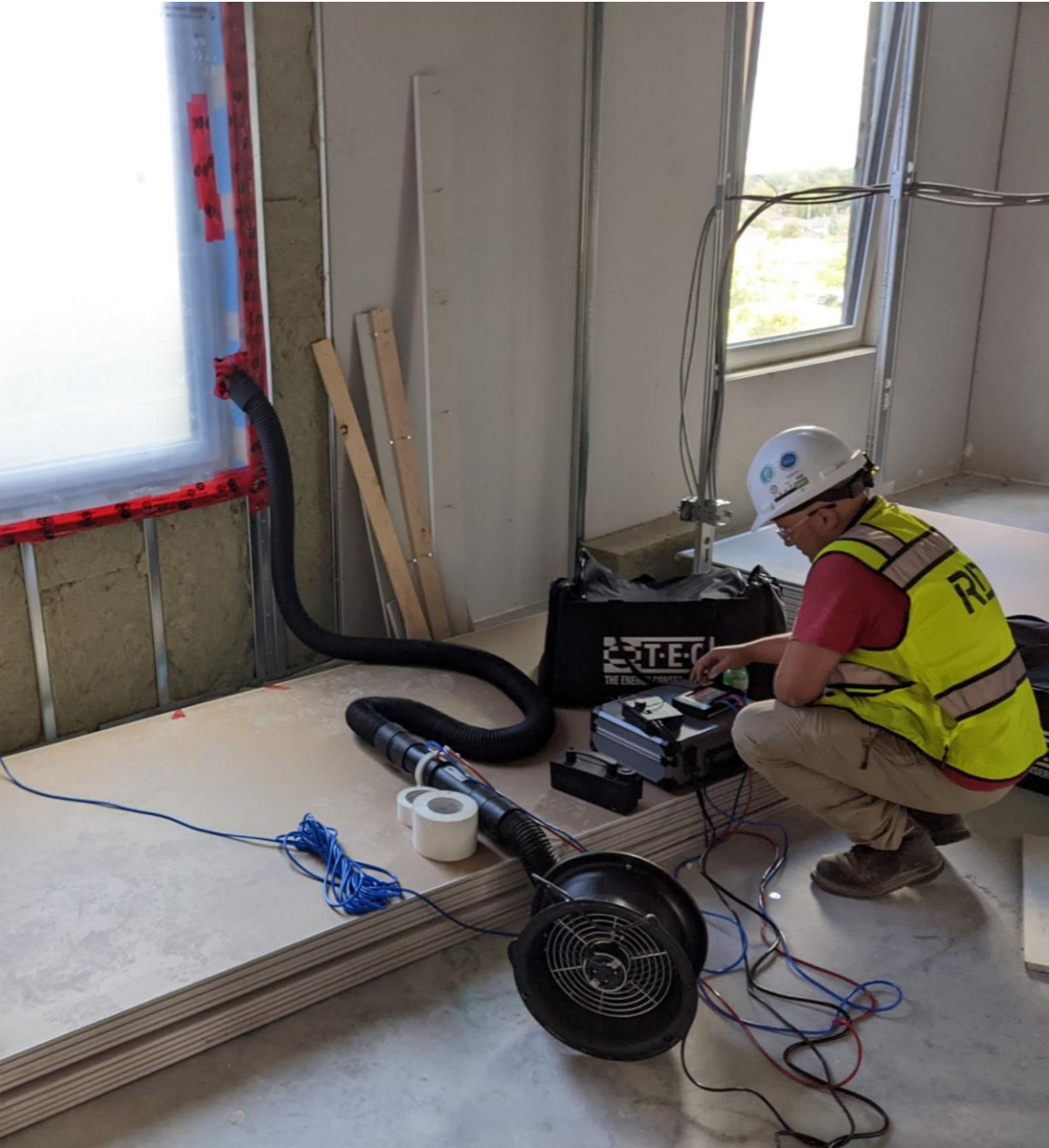
Window installation air leakage testing
