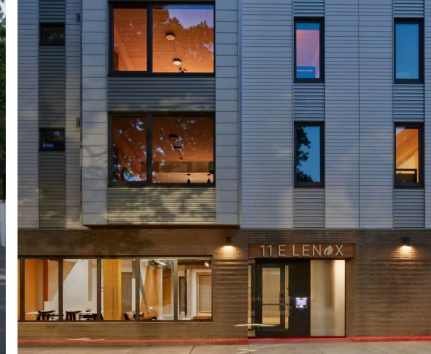
11 E. Lenox Street Boston MA Haycon Construction
