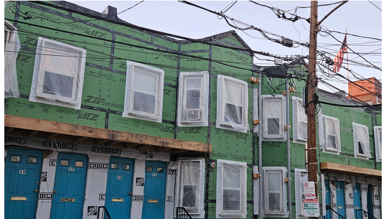
Hano Homes, Passive House Retrofit Project
