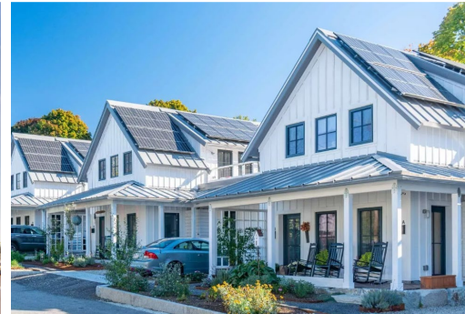
Hillside Center for Sustainability Newburyport MA Hall & Moskow
